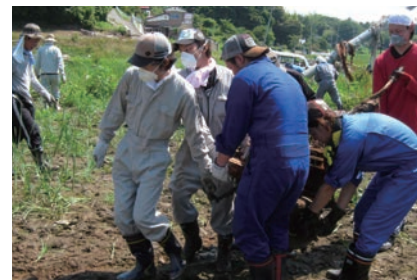
JSR volunteers participate in restoration activities in earthquake-affected area.
